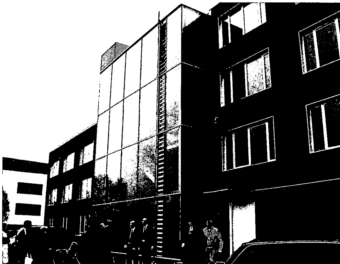
Foto 7. Fachada norte edificio Balanced Office Building, Aachen
